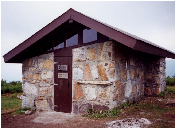
The completed shelter after three weeks of work. Chestnut Knob is the high point of PATH’s section, both literally and figuratively. The shelter was also featured in a recent book about notable shelters on the AT.
