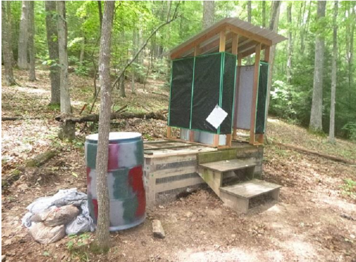
The Jenkins Shelter Privy with two holding bins and recently installed enclosure. Note the wood shavings barrel and grocery sacks full of shavings carried in by hikers. Photo by Herb MacDonald.
